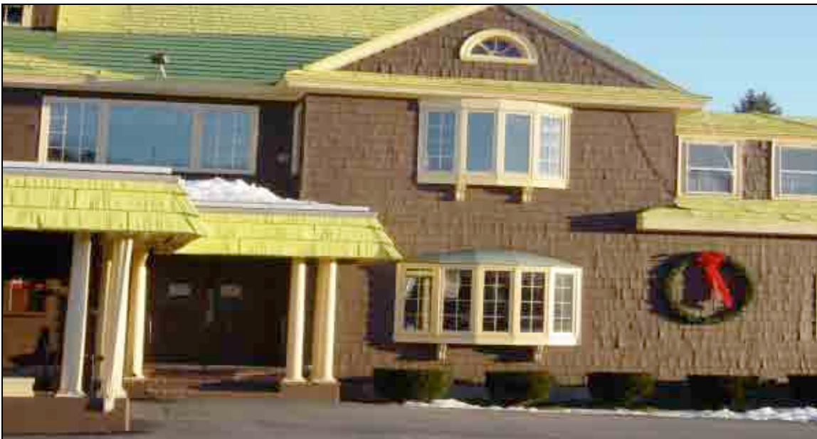
The gables, bay windows and shingle siding contribute to the traditional New England appearance of this building.
